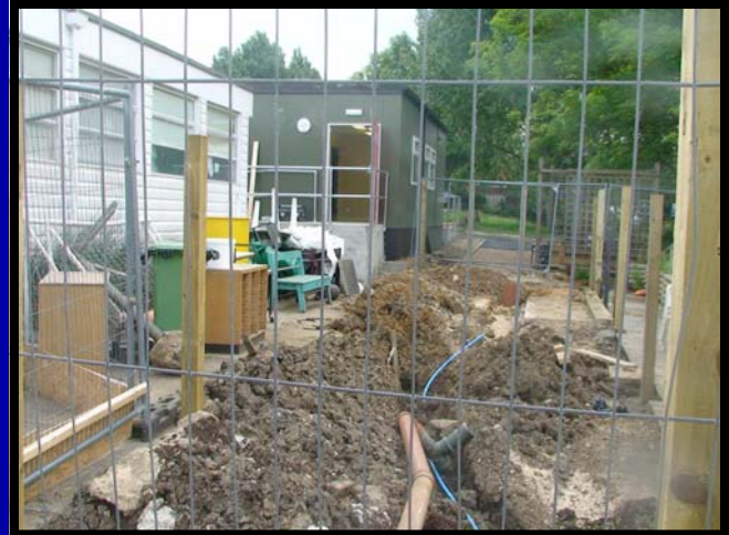
New pipes are laid for drainage
