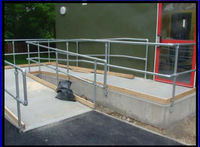
The mobile is now fitted with a ramp for wheelchair accessibility
